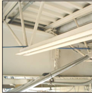
Ceiling Dust Removal
