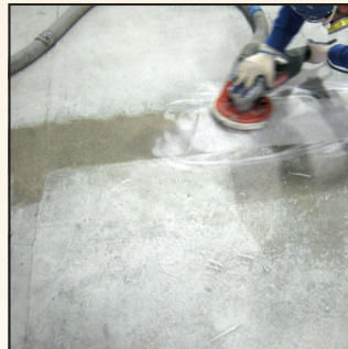
Slab Grinding
